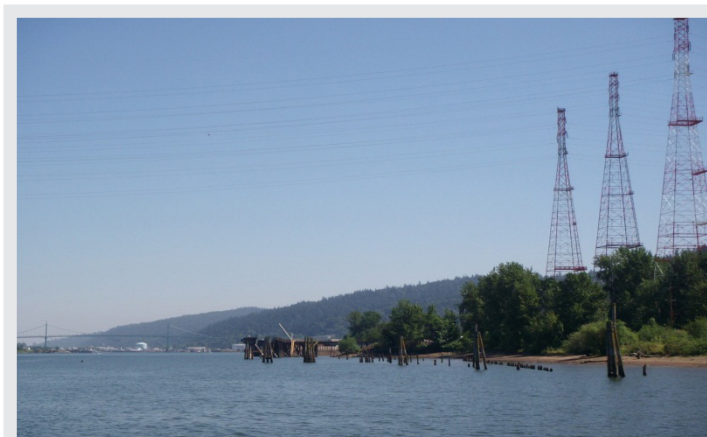
Left: These high voltage electrical transmission towers are built on a river bank in the Critical Energy Infrastructure (CEI) Hub susceptible to lateral spreading. (DOGAMI photo)
