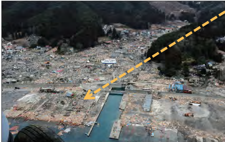
An aerial view of damage to Otsuchi, Iwate prefecture, Japan on March 15, 2011, after the magnitude 9.0 Tōhoku earthquake and subsequent tsunami devastated the area; 11.6% (1,378 people) of the exposed population were killed or are missing. In Iwate prefecture, 4,667 were killed and 1,363 remain missing. (U.S. Navy photo by Mass Communication Specialist 3rd Class Alexander Tidd/Released)
