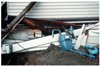
Houses don't need to collapse to be evacuated. This house shifted off its foundation in the 1989 Loma Prieta, California quake and now all the utilities are disconnected. Photo: H. G. Wilshire, USGS
