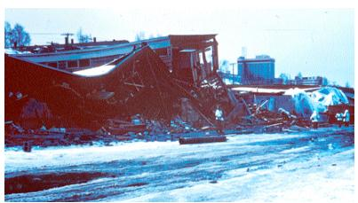
Warehouses at the toe of the Fourth Avenue landslide in Anchorage in 1964 were destroyed by compressional buckling and foreshortening. Much of the supply of food and drink for the city was stored in these buildings. Photo: USGS
