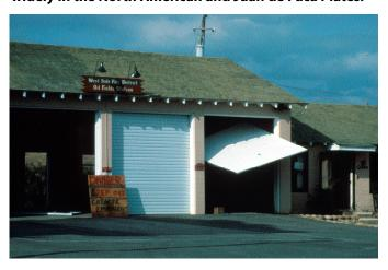
In the 1983 Coalinga, California earthquake, this fire station was badly damaged (note the skewed door). If rescue equipment can't get out of the station, it can't be used when needed after an earthquake. Photo: M.G. Hopper, USGS
